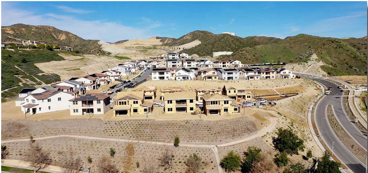
Tesoro Highlands under construction, July 2024
